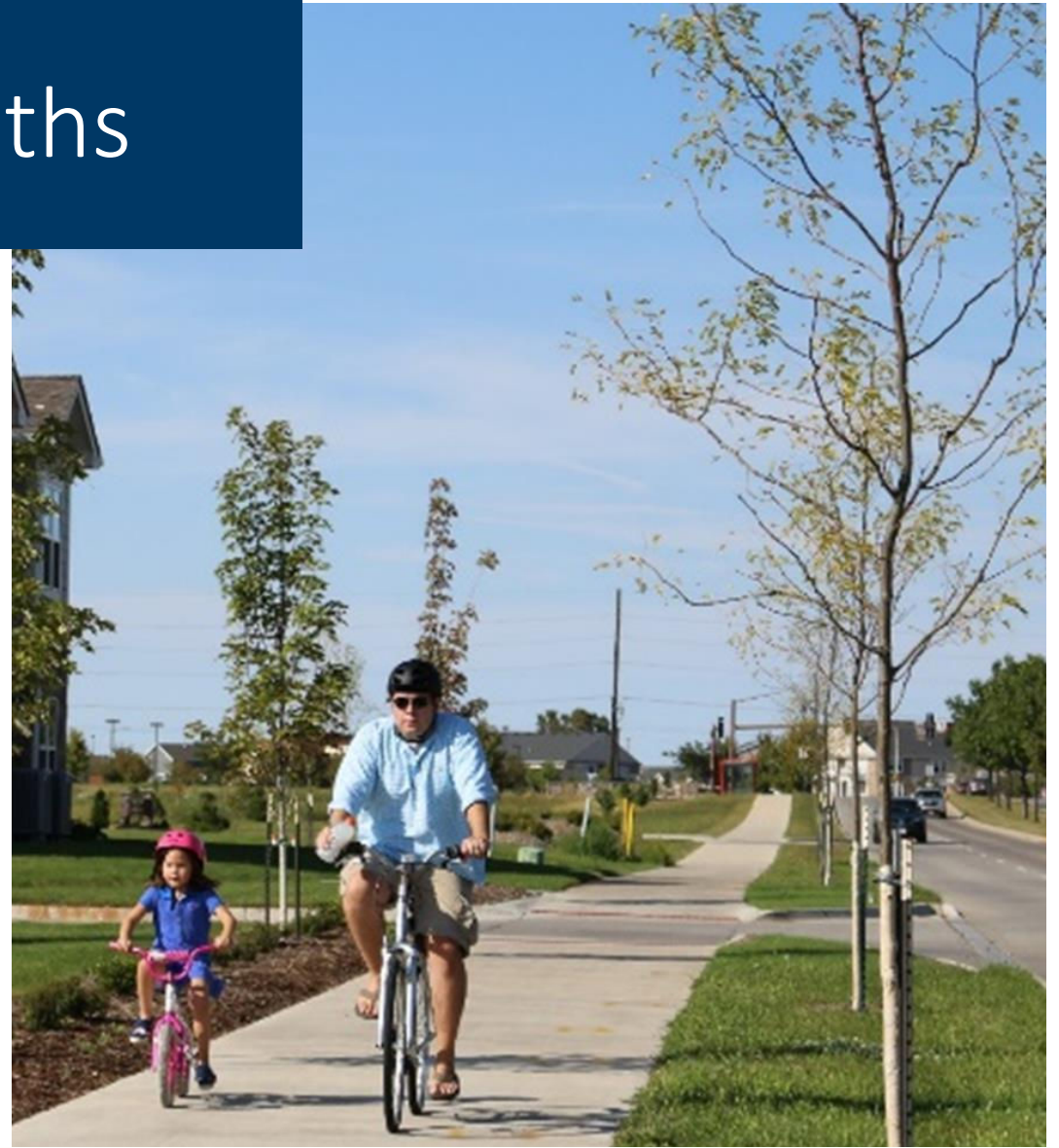
Sidepath trails: bidirectional shared use paths that run parallel to the roadway. Roadway intersections and driveway crossings require consideration to protect trail users
