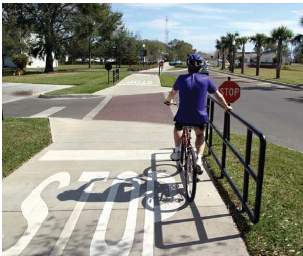
Enhance trail crossings in New Ulm with high-emphasis markings and a rail upon which bicyclists can lean, such as this part of the trail through Winter Garden, FL.
