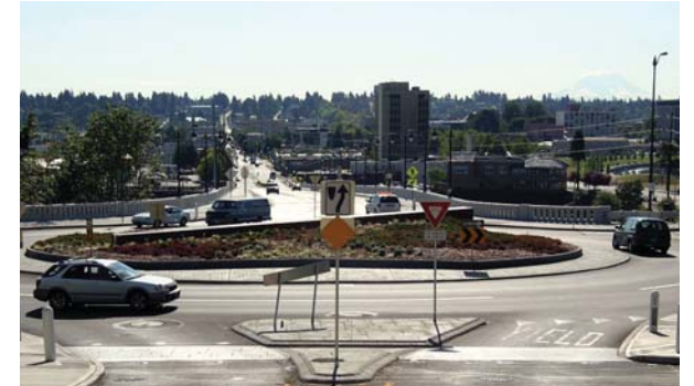
The modern roundabout above, in Olympia, WA, is on a sloped street, like Center, and serves as a traffic-calming gateway into an important part of town.
