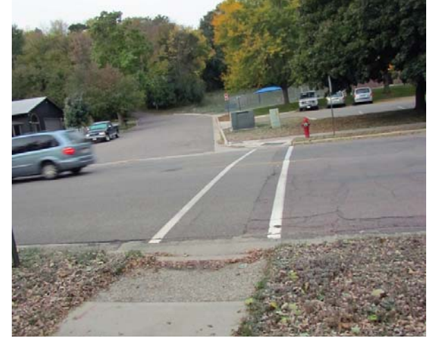
This crosswalk provides very little cue to drivers that they should expect to yield to people crossing here.
