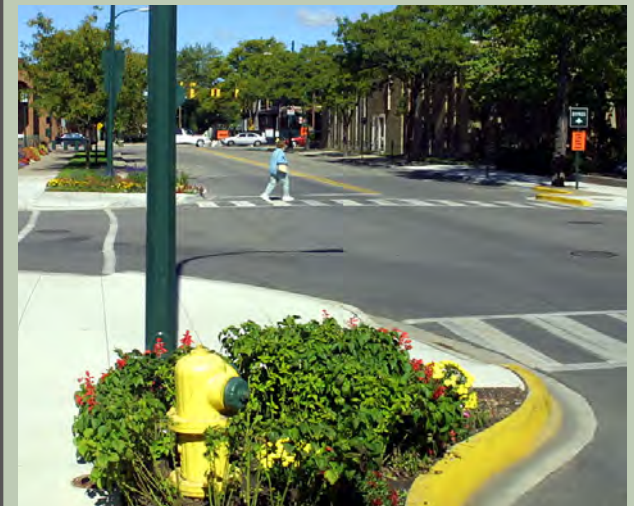
A curb extension in Birmingham, AL shortens the crossing distance for pedestrians.
