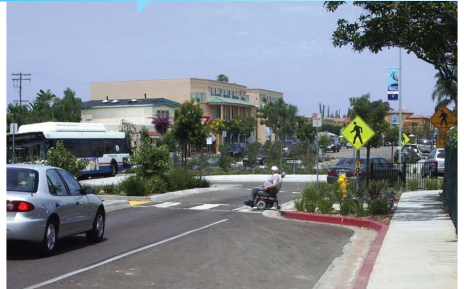
This single-lane roundabout in San Diego carries about 25,000 vehicles per day, far more than the volume of Center, while enhancing safety for all. Pedestrians cross only one lane at a time, and drivers yield appropriately due to lower vehicle speeds.
