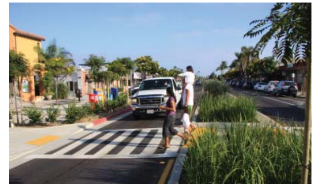
Roundabouts make crossings easier because the pedestrian crosses one leg at a time. The lower vehicular speed increases yielding behaviors by drivers. To assist visually impaired pedestrians, pavement markings can be positioned to provide an auditory clue that cars are entering and existing the intersection.
