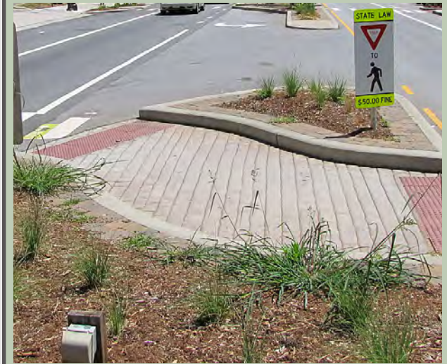
Pedestrian refuge islands buffer pedestrians from traffic, allow crossing in stages and angle pedestrians correctly to face traffic.
