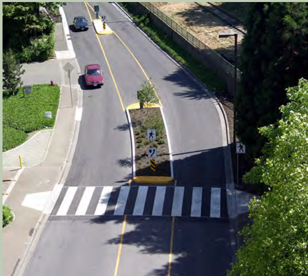
Crossings must be located where there is a strong desire to cross and sight distances are good.
