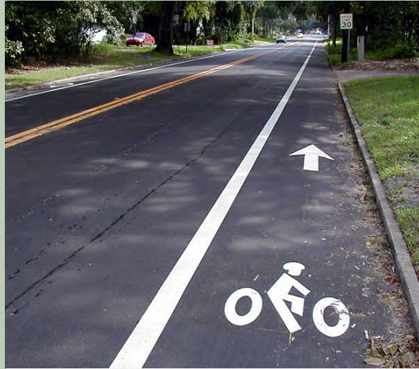
Bold striping and markings remind drivers that bicyclists should be expected on the road.
