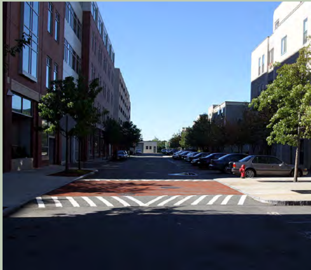
A raised mid-block crossing in Cambridge, MA helps motorists see pedestrians in deep shadow.
