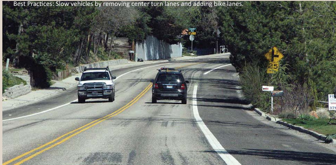
Best Practices: Slow vehicles by removing center turn lanes and adding bike lanes.
