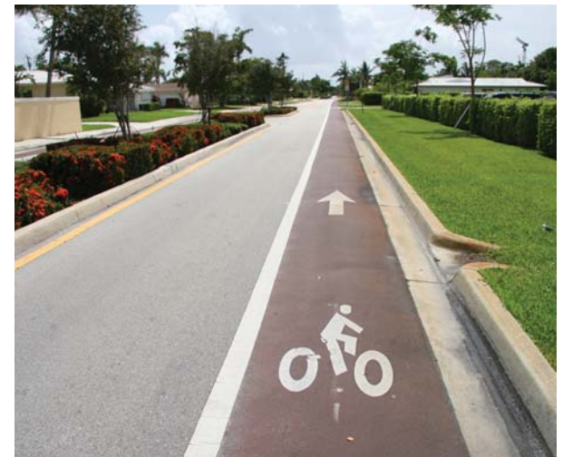
In Boca Raton, FL, colored bike lanes create even more visual delineation of space for bicyclists. The narrower vehicle lanes also tend to help calm traffic.
