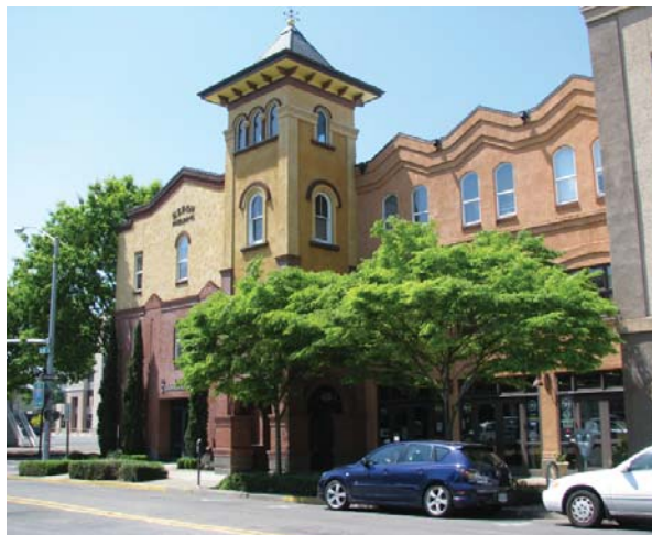
A mixed-use infill project in Eugene, OR.
